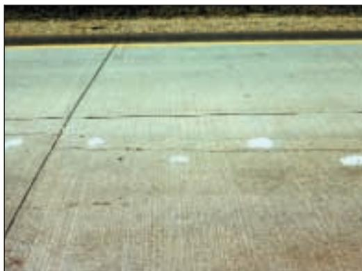
6. Completed cross-stitching on longitudinal crack.
